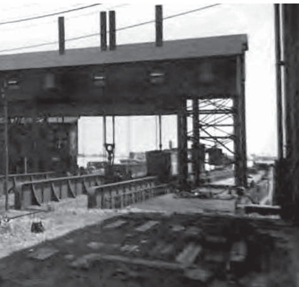
A PRRC composited panoramic photograph documents the condition of the Greenville Yard transfer bridges circa 1940, several years prior to the addition of Bridge 9. This northeastward view was reproduced in 2011 HAER documentation of the Greenville Yard Transfer Bridge System and Freight Operations (Hayden 2011).
