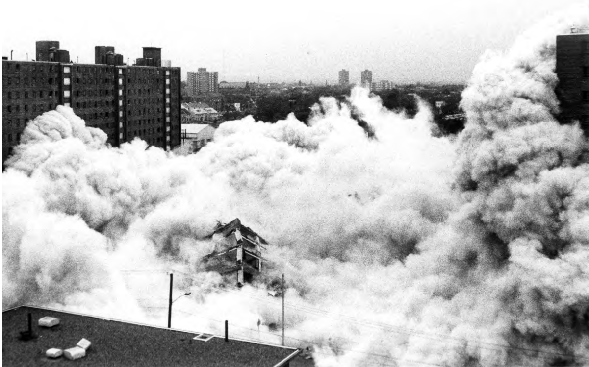
Demolition of Scudder Homes projects, 1987. Courtesy New Jersey Newsphotos
